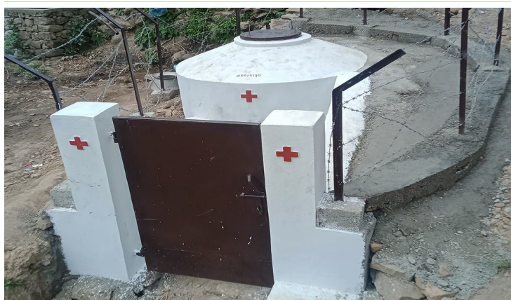
Ferrocement Tank being constructed in Tinau RM, Palpa (PC: Krishna Prasad Subedi, NRCS, HQs)
