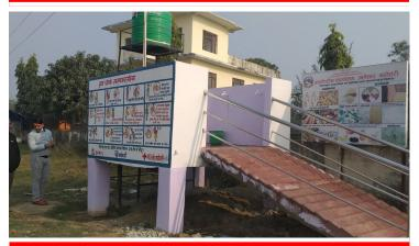
Raised hand pump and hand washing station at point of entry (PC: NRCS Mahottari)
