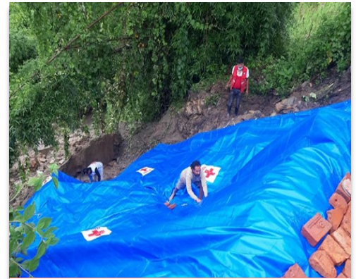
Tarpaulin laid to stop the landslide
