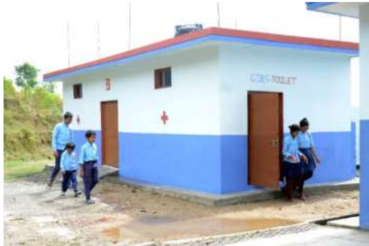
Nepal Red Cross Society has supported the construction of child gender disabled (CGD) friendly toilets in Shree Mahindra Lila Secondary School, Gorkha district.
